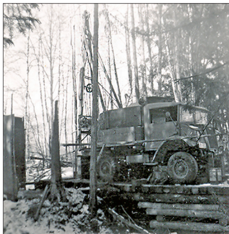
A drilling rig at the soda spring in Mara in 1953 when the Gas-Ice (Canada) Corporation Limited was looking for carbon dioxide in 1953. [MS99-230]
