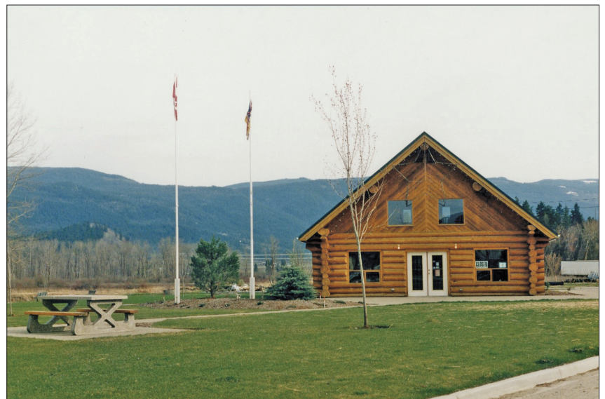
The Enderby & District Chamber of Commerce Building, 700 Railway St. in 1996. Note the size of the tree to the left of the building. [edms 5347]
