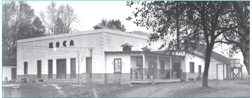
NOCA in Enderby in December 1939 after a fire destroyed the top floor and the building renovated. [edms 0024]
