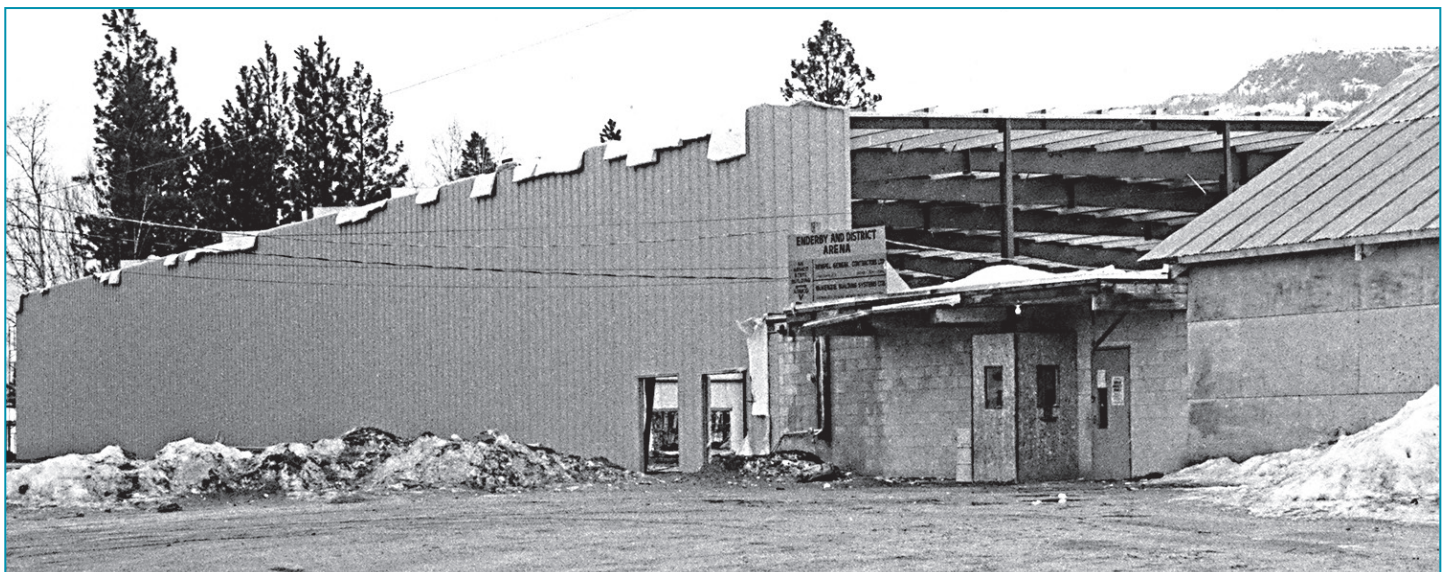
Construction of the new Enderby Arena in 1975. [edms 3685]
